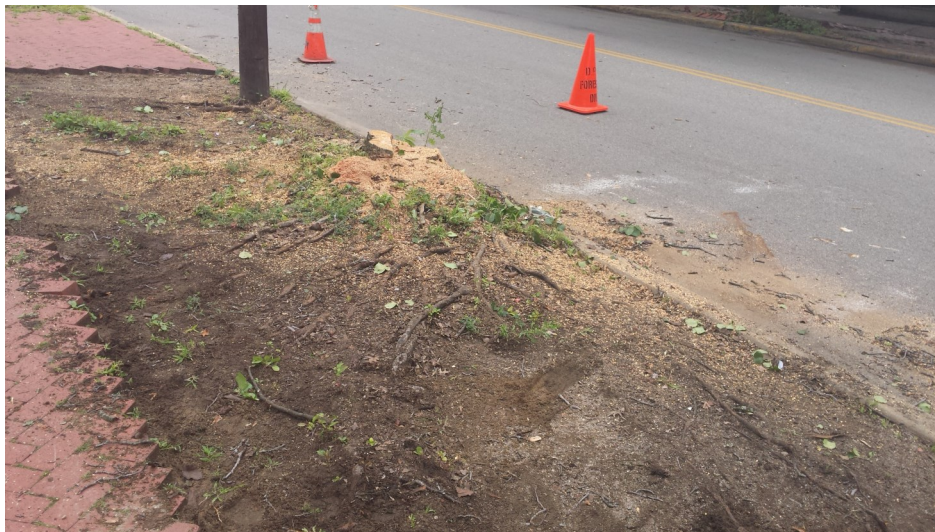
Example of sidewalk deconstructed and existing stump/root system
