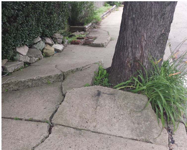
Common sidewalk damage throughout Manchester
