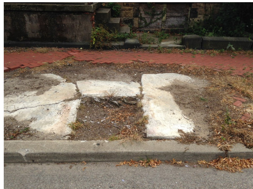
Concrete and red brick sidewalk construction in Manchester
